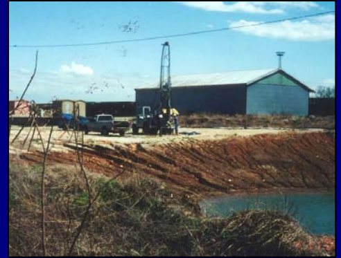
Installation of soil borings and collection of soil samples from the banks of a lagoon.
