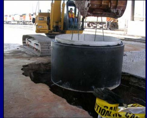
Lift station installation
